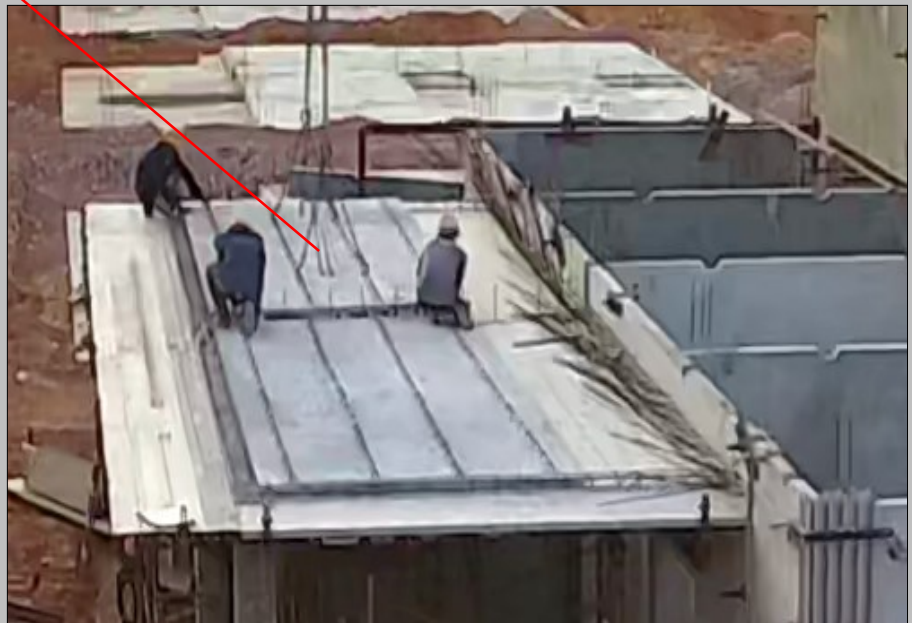
- Precast half-slab installation
