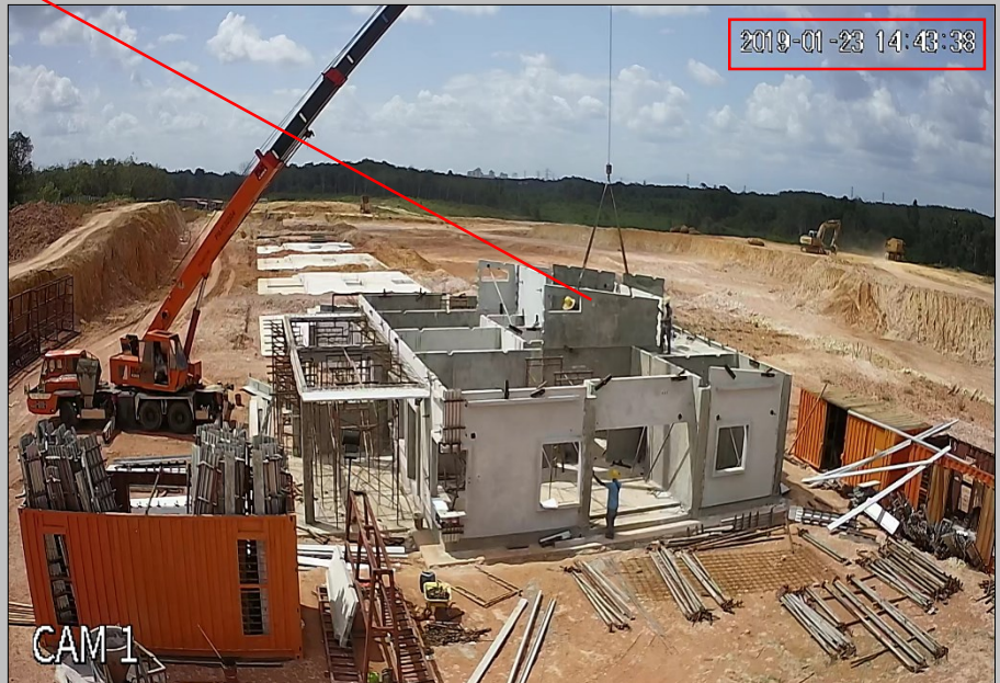
- Precast wall panel installation
